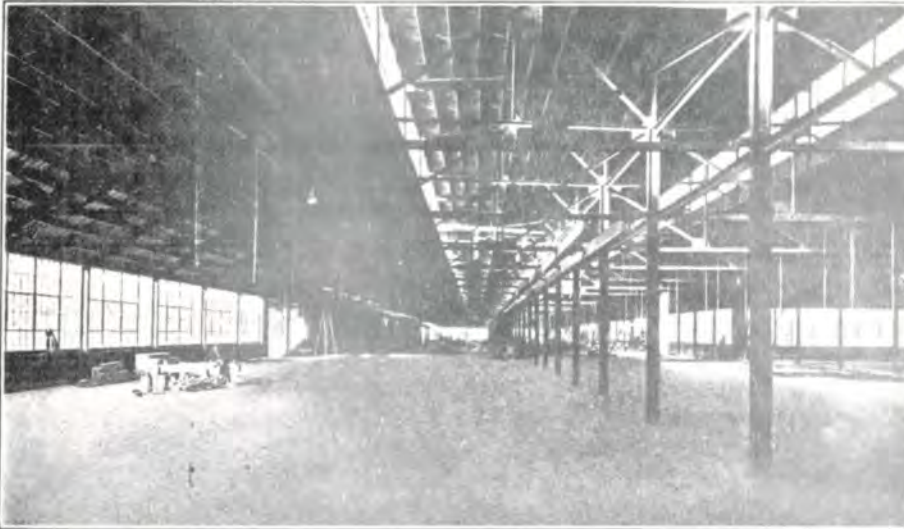
Interior of new Central Building before equipment was installed
