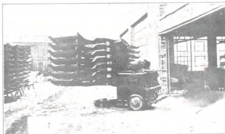
One man with device can handle 250 frames easily a day
