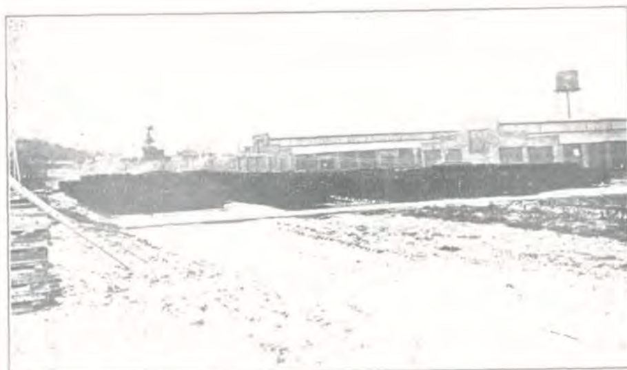
Frames piled on metal horses so they can be picked up by device shown in picture above
